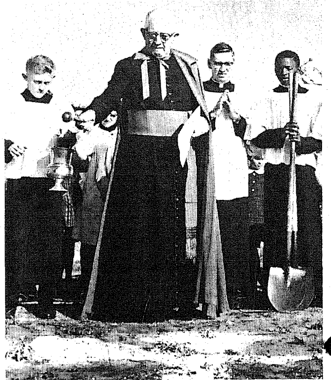
NEW CHURCH of St. George will be constructed in Fort Lauderdale where MSGR. JOHN J. O'LOONEY, pastor, St. Anthony parish, officiated at ground-breaking ceremonies. FATHER LAURENCE CONWAY, right, is pastor.
