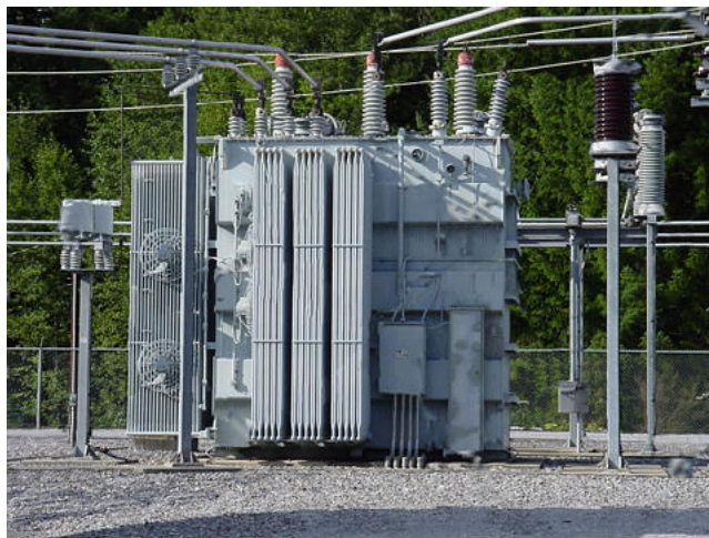
Figure 9.20: Substation transformer.
