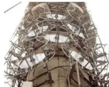
FM circularly polarized antenna system built as an array of back-cavity unitary radiators
